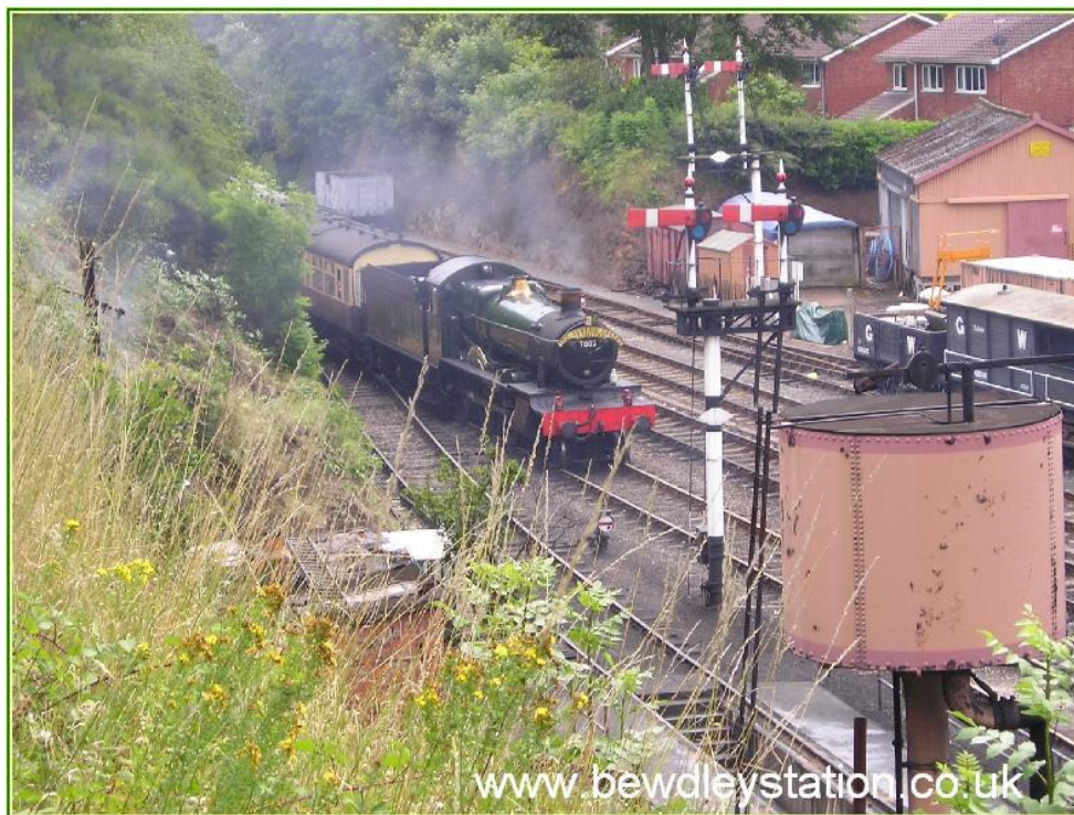
An unusual angle to view the southern end of the station from, and one which is not normally accessible. 7802 Bradley Manor is entering Platform 3 with The Severn Valley Limited dining train. The MPD locomotive inspection pit is seen in the foreground whilst in the background part of the carriage works is visible
