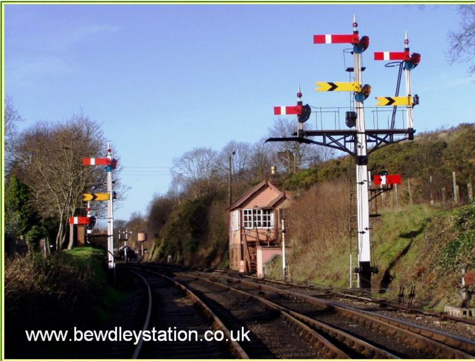
Bewdley South Signal Box showing some of the signals associated with the Stourport junction. The signals on the right hand bracket control access to Platforms 1 and 3, plus the Rock Siding and Down Goods Yard for trains from Kidderminster, whilst the small bracket on the left of the alignment controls access to Platform 1 and the Down Goods Yard for trains from Stourport. The highest yellow signal is the Bewdley North Up Distant and can be operated By North Signal Box when the home signal is pulled off. The other distant signals are fixed. Photograph By A.Coley
