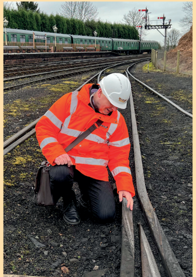
Track is worn and cracking
